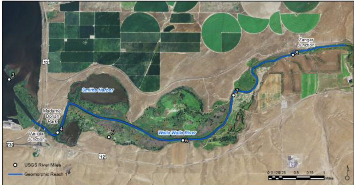
Figure 3-1. Aerial View of Geomorphic Reach 1
